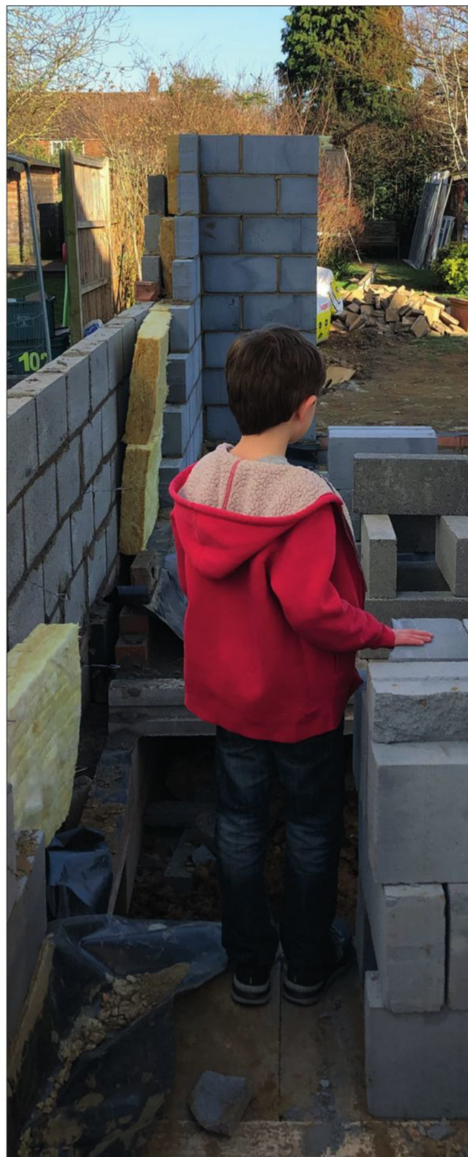
Above: Edward Lacey, 7, checks progress on the new extension.
